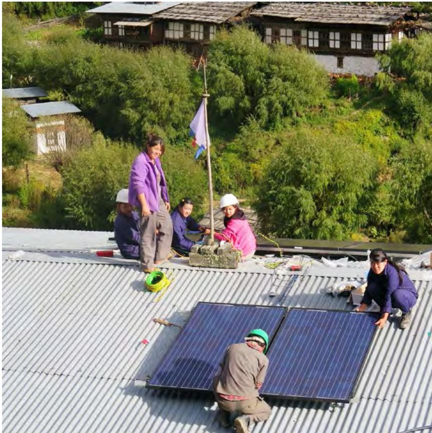
Trainees installing solar water heating system on the shagor roof
