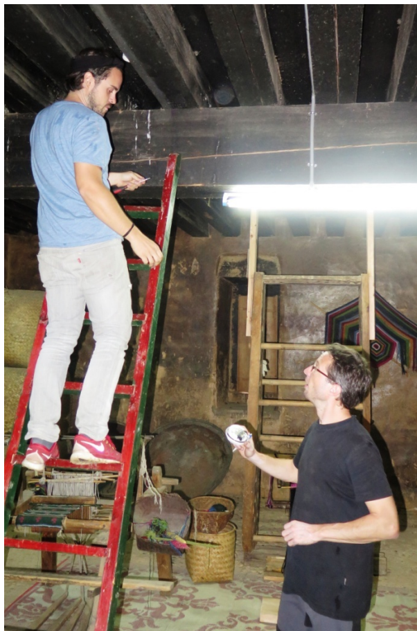
Installing smoke detectors for fire alarm system
