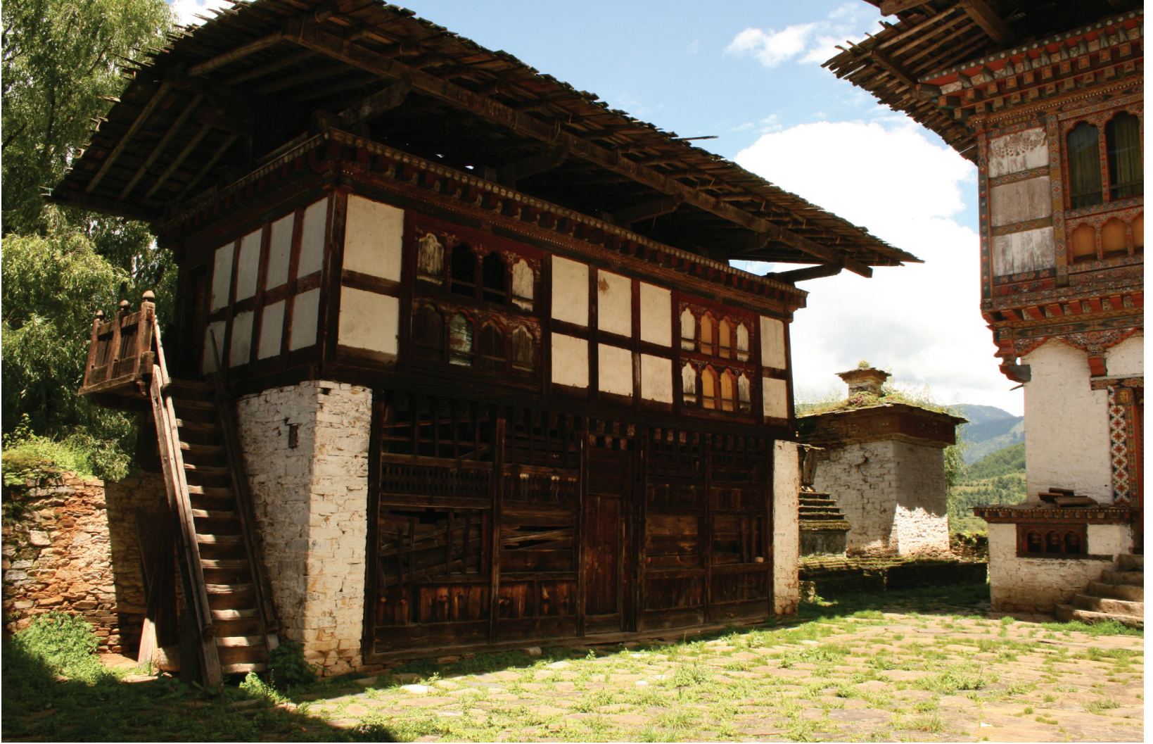
FIGURE 5.2: THE CHAMKHANG TODAY, THE ONLY BUILDING THAT SURVIVED THE EARTHQUAKE OF 1897
